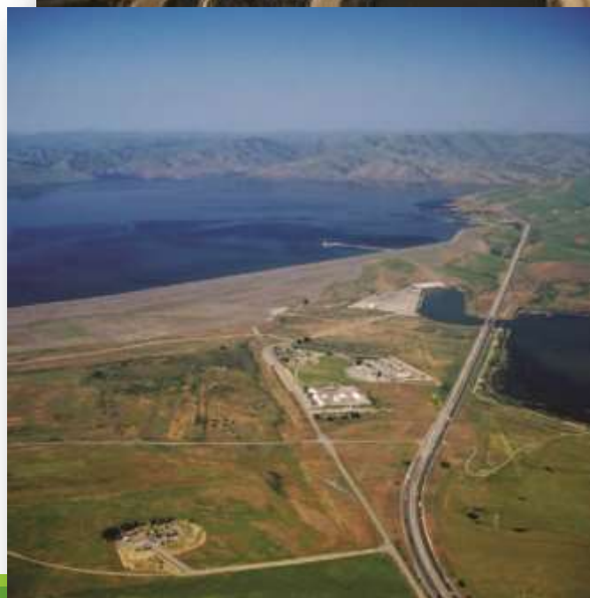
Harvey O. Banks Pumping Plant
